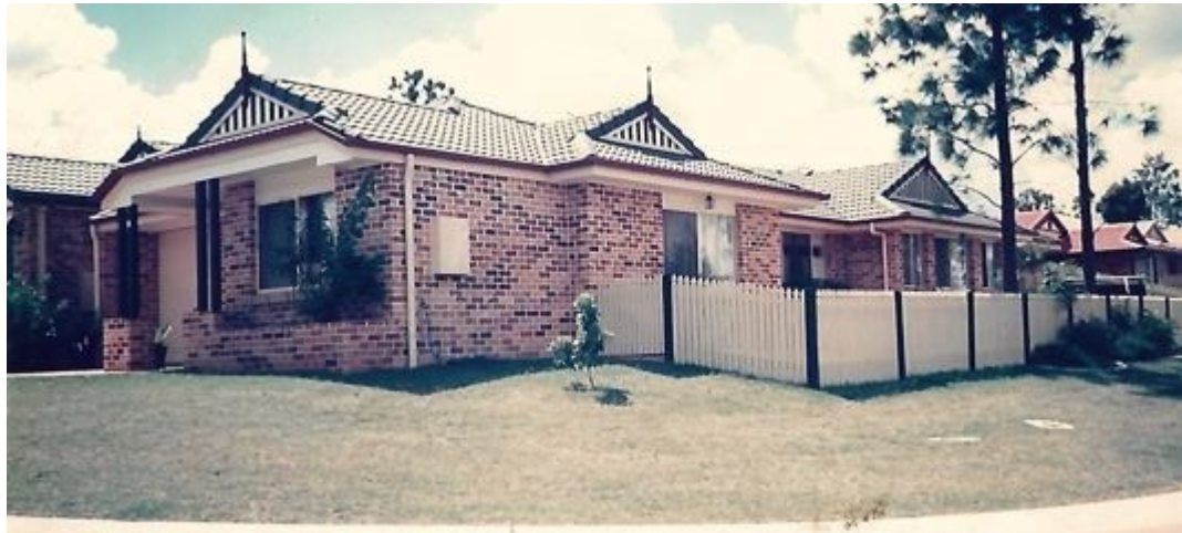
18 Evergreen Place, Forest Lake, Queensland - at time of purchase (no garden)
